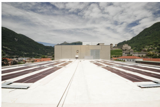
Figure 3: The thermal behavior of the “Scerri” plant will be compared with the “CPT” plant, different producers and technology (single vs. triple-junction a-Si modules).
